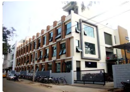
Dynamatic Hydraulics™, Unit II
