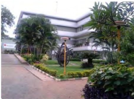
Dynamatic Hydraulics™, Unit I
